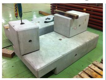
The shielding has been successfully assembled in the PS and is now ready for final installation in SS15. Note: Block 1 (Base block) has a lifting point on the geometric centre of the block but due to the removal of some of the block (for Bus bar clearance) the centre of gravity has shifted. When this block is handled it is recommended to place blocks 6 and 7 on the block above the bus bar location to compensate for the change in C of G. This will allow the transport of this block in a horizontal
