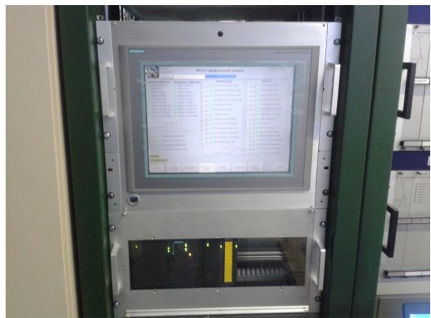
local HMI and master PLC (Siemens S7-317F)
